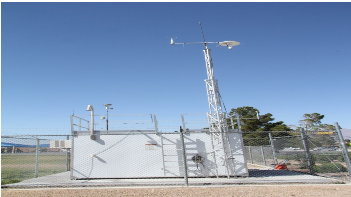
Figure 125. Joe Neal Monitoring Station (EPA 32-003-0075)—Street View.
