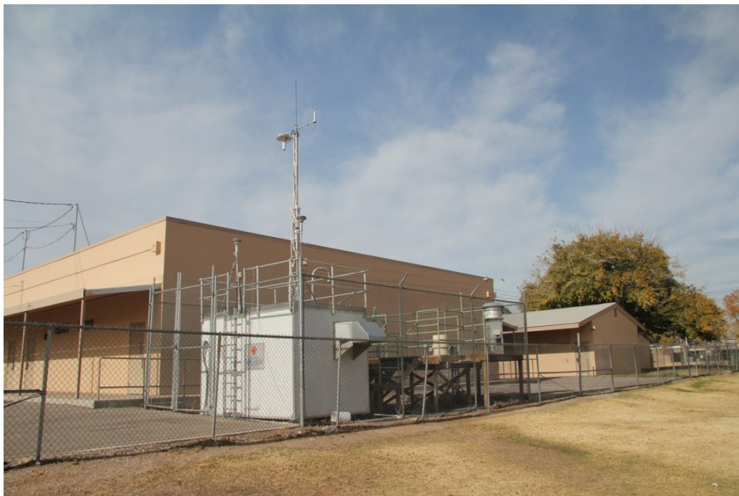
Figure 120. J. D. Smith Monitoring Station (EPA 32-003-2002)—Street View.
