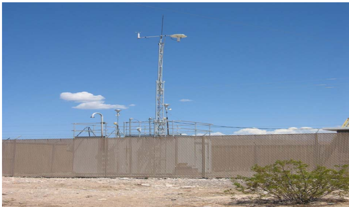
Figure 145. Jean Monitoring Site (EPA 32-003-1019)—Street View.
